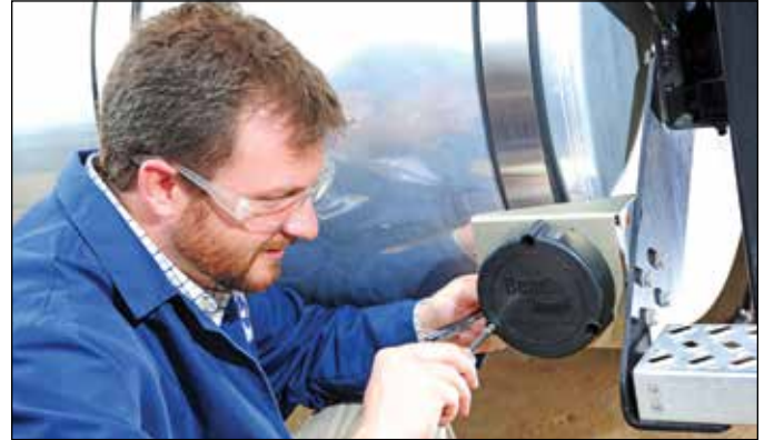
FIGURE 5 - INSTALLATION OF SENSOR
